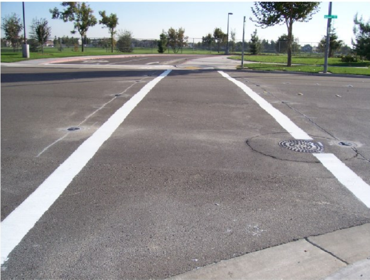
Fixtures Placed In Base Cans
