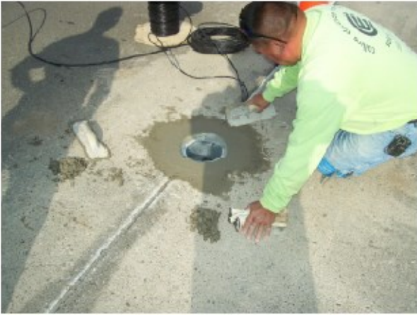
Base Can in Concrete
