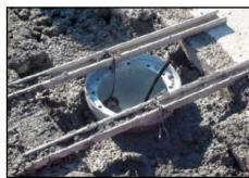
Mounting Jig Attached to Base Can
