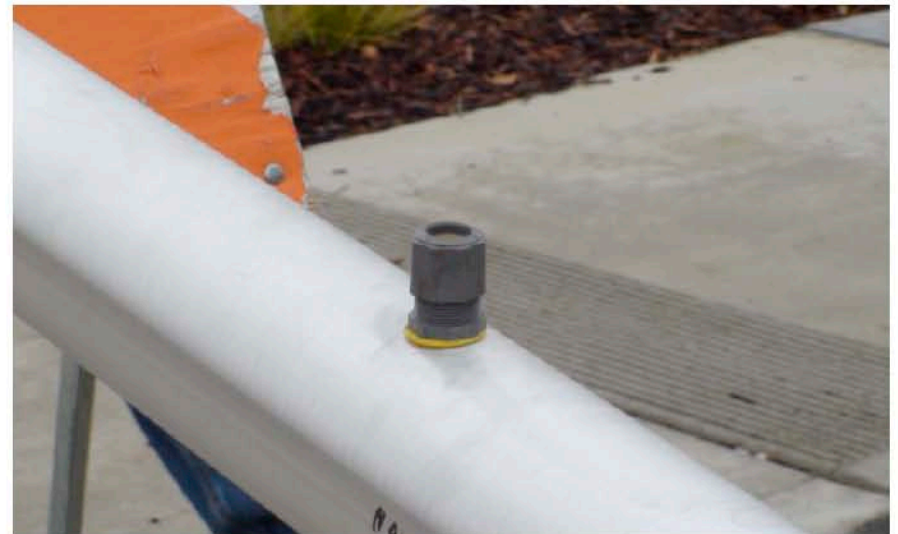
27. Waterproof Electrical Fittings are attached to the Pole for Flashing LED Sign Cabling.
