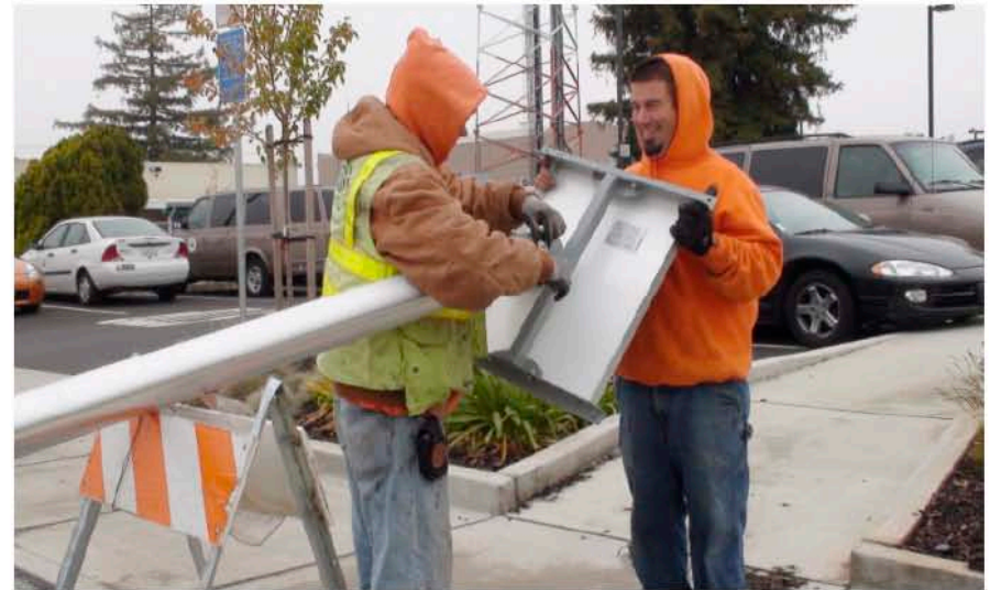
29. Solar panel is then attached to the pole.
