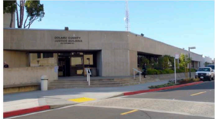
47. Solano County Justice Building.
