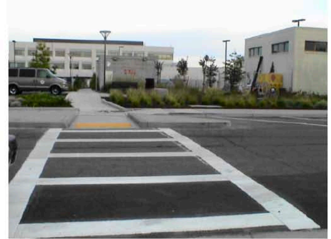
3. Crosswalk site before system installation.
