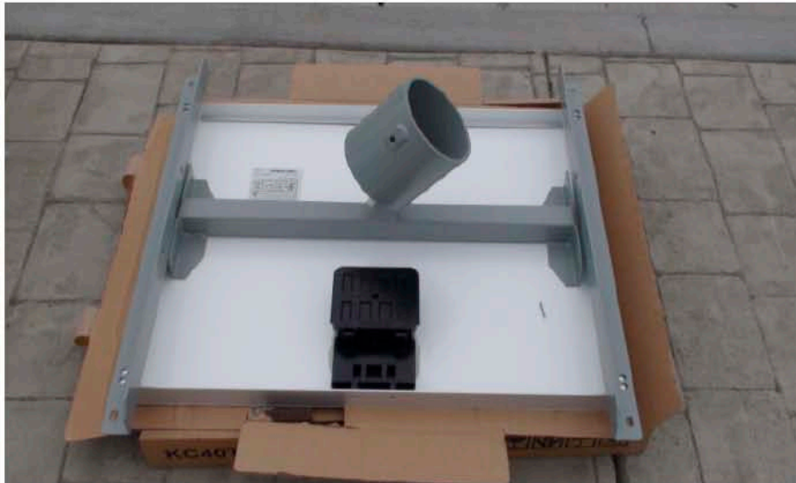
28. Pole mounting hardware is attached to the solar panel.
