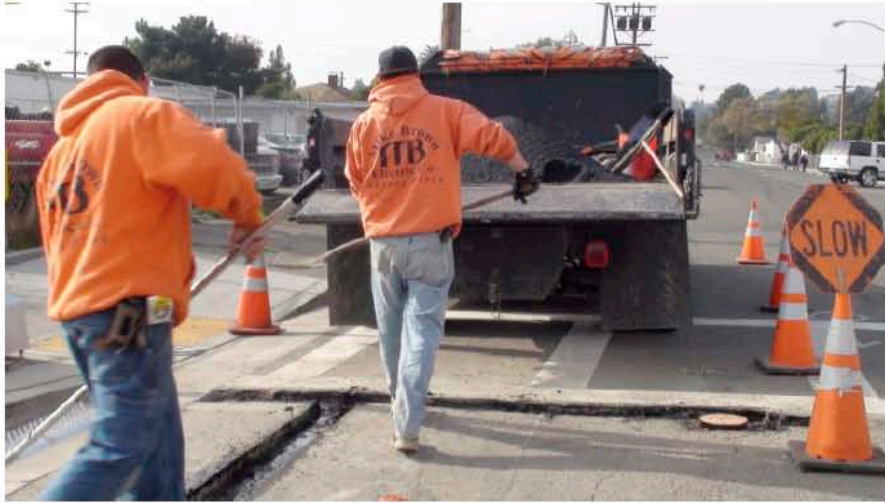
38. After all street cabling has been completed; asphalt is shoveled into the trench and leveled with a rake.
