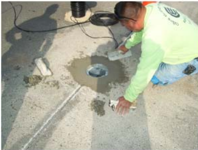
Base Can In Concrete
