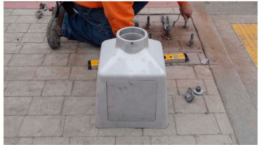
25. Pole base shown with access door positioned towards the side walk.
