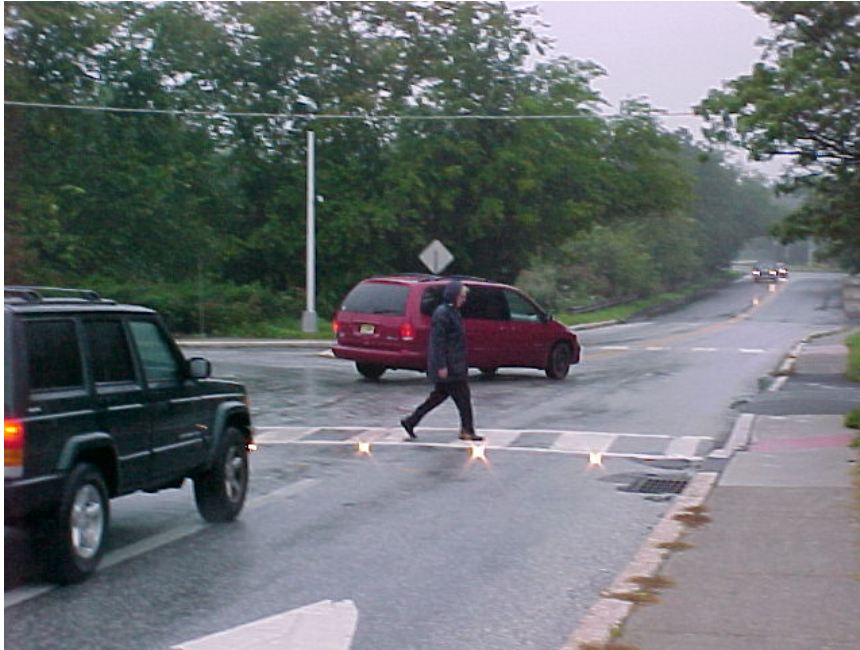
FIGURE 5 Crosswalk 1 with the in-pavement flashing warning lights installed and operating.
