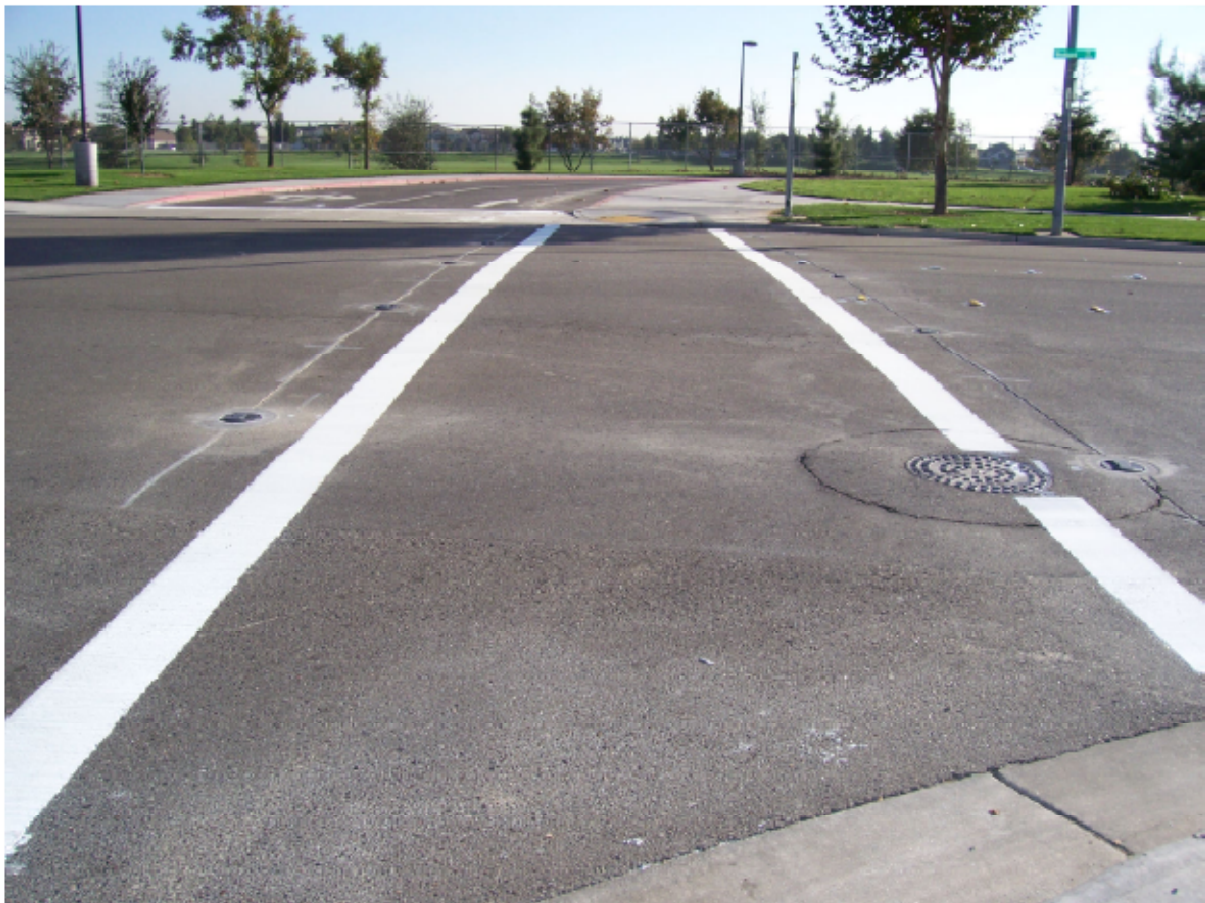
Fixtures Placed In Base Cans
