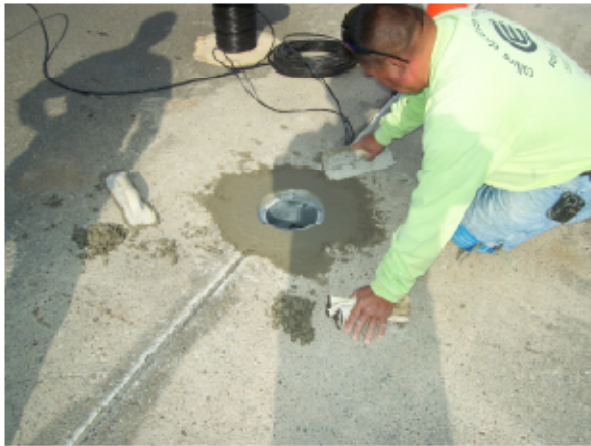
Base Can In Concrete
