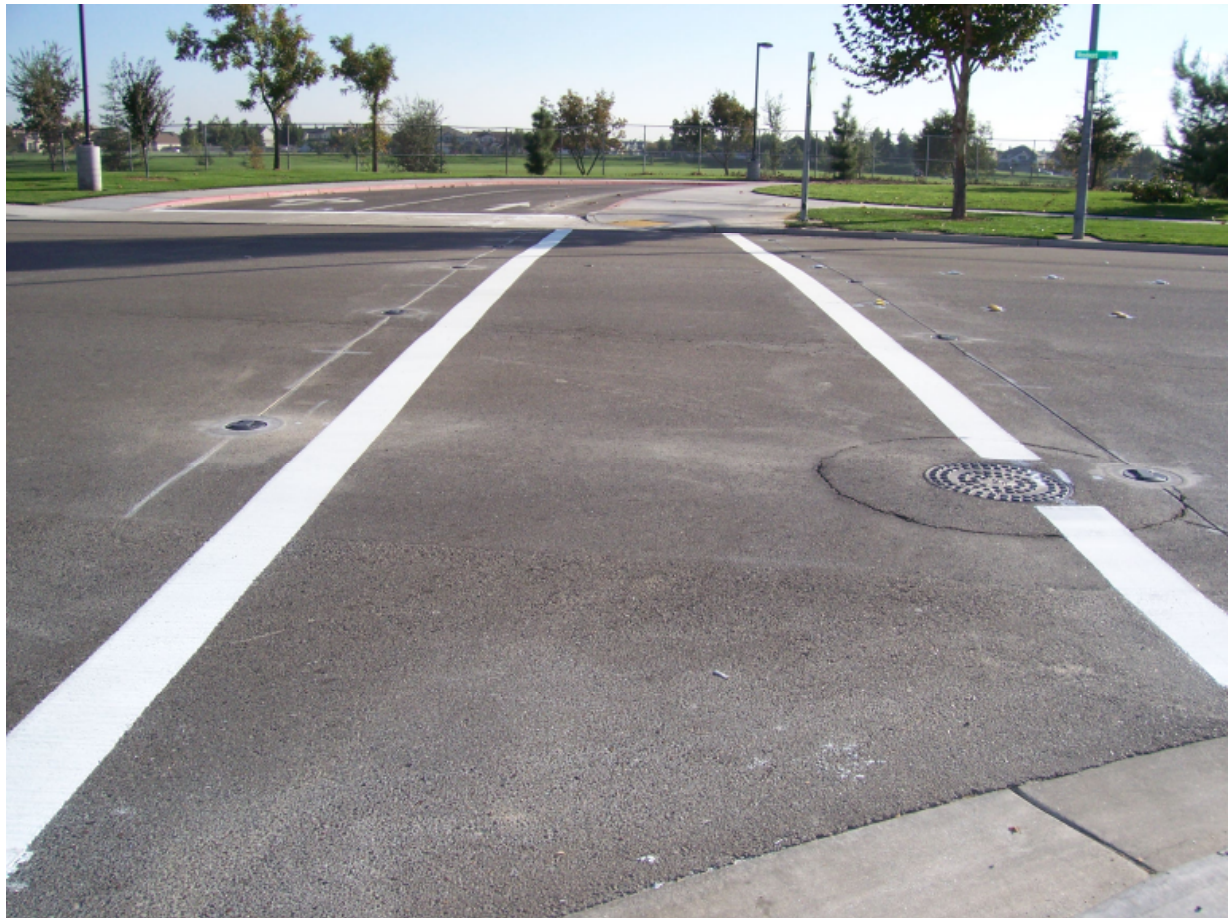
Fixtures Placed In Base Cans
