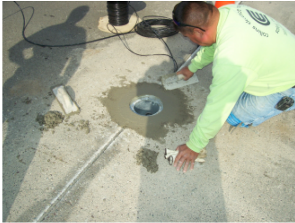
Base Can In Concrete
