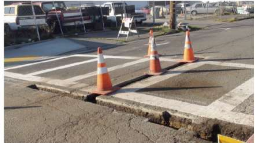
11. Trench is now completed and ready for Installing the Base Cans and Conduit.
