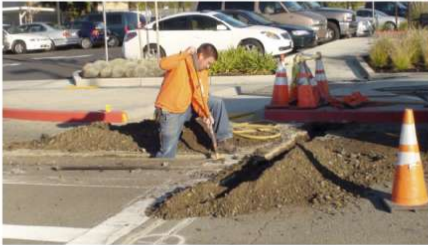
10. The final phase of the trenching is completed with the use of a trench shovel.
