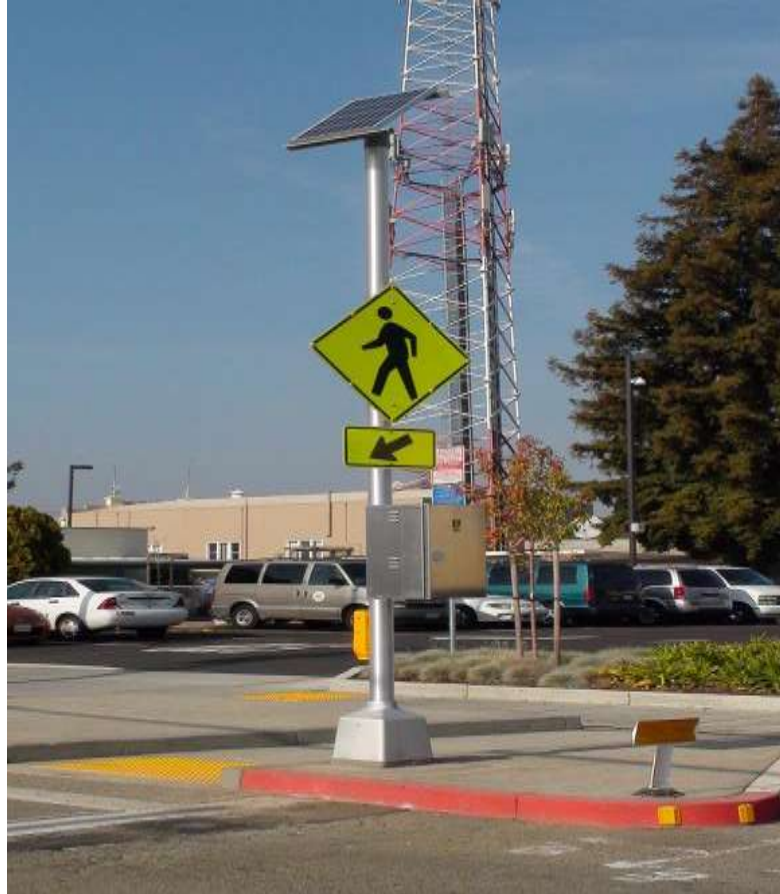
50. View of pole assembly showing the solar panel facing True South , flashing LED pedestrian sign, crosswalk arrow sign, and TS1000 system enclosure.
