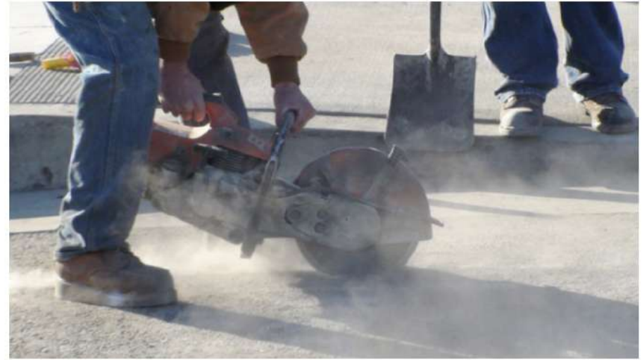
7. A dry cut is then made to cut along the outline of the trench.
