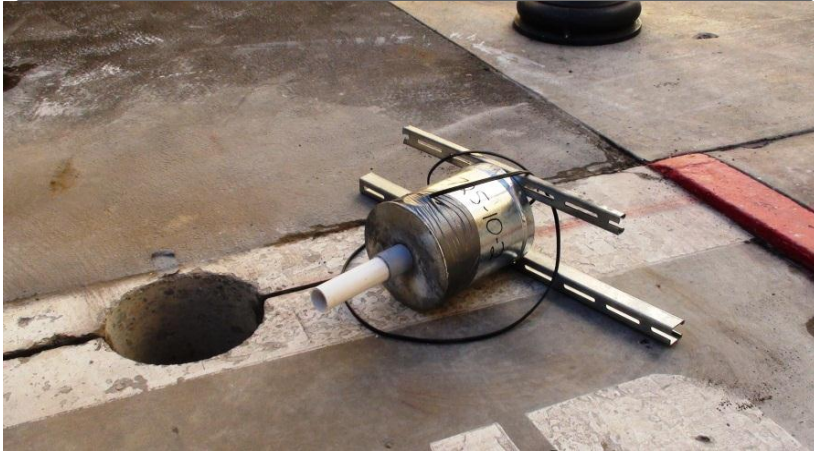
Figure 21: Mounting Jigs are Bolted to the Base Cans to Hold Base Can Flush with the Pavement and Field Wiring is Routed Through Base Can
