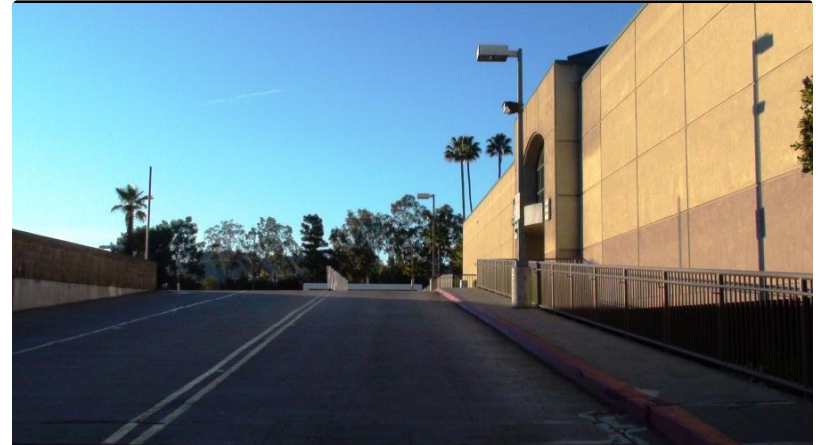
Figure 6: Ramp to Second Level Presented A Crosswalk Visibility Issue
