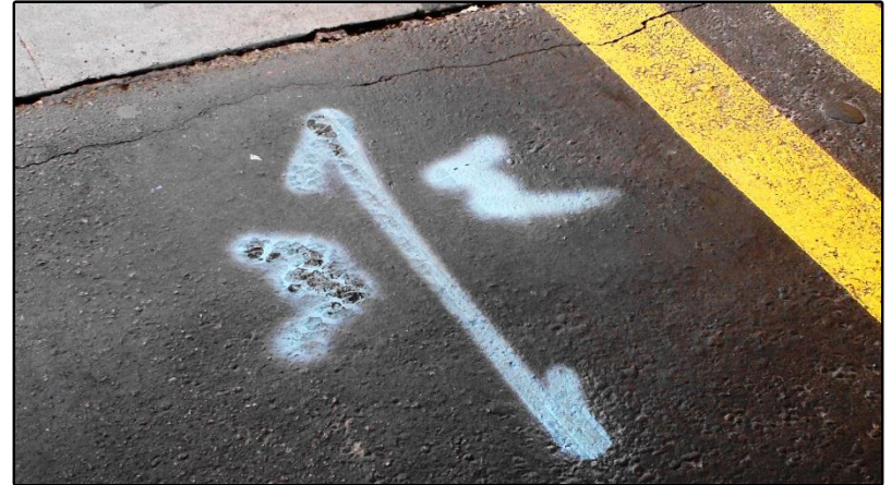
Figure 10: APWA Color Code, Blue = Water Line
