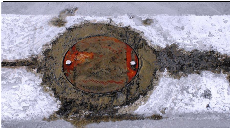
Figure 23: After Concrete is Cured the Mounting Jigs are Removed. The Plywood Covers are Left on Until the Fixture is Installed
