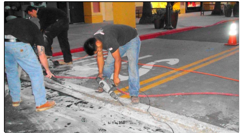
Figure 16: A Channel, Approximately \frac{1}{2} " Wide and 3" Deep is then Chiseled Away between the Saw Cuts
