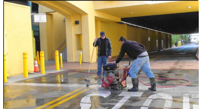
Figure 14: The Saw Cuts Continue Across the Length of the Crosswalk, Crossing all Fixture Locations
