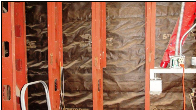
Figure 31: Controller Enclosure Location Area Cleared and Prepared for Mounting Back Panel
