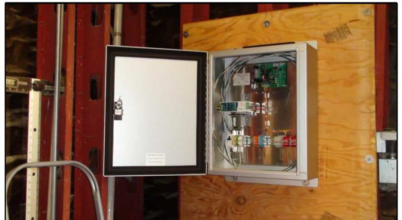
Figure 32: Back Panel Bolted to Wall and Controller Enclosure is then Bolted to the Back Panel
