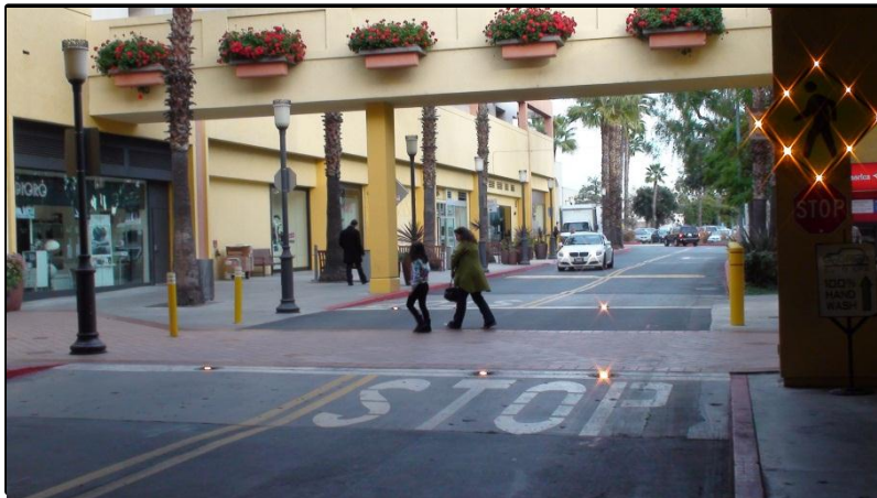
Figure 35: Warning Light System Protecting Pedestrians During the Day
