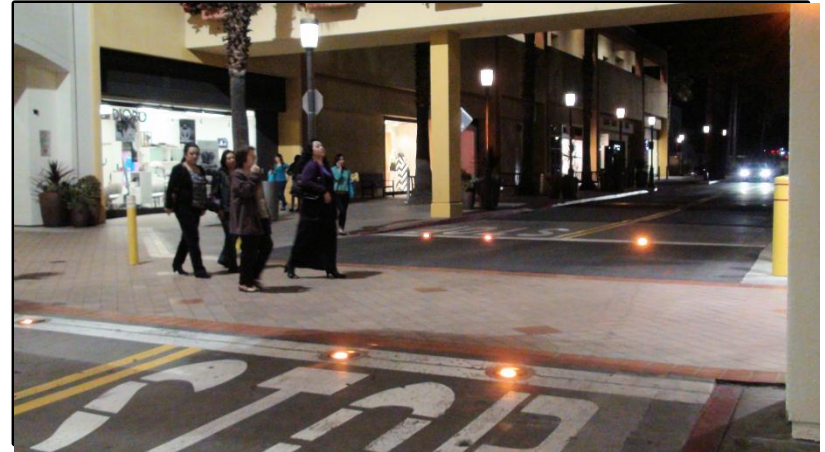
Figure 38: Warning Lights are Clearly Visible to Drivers at Night
