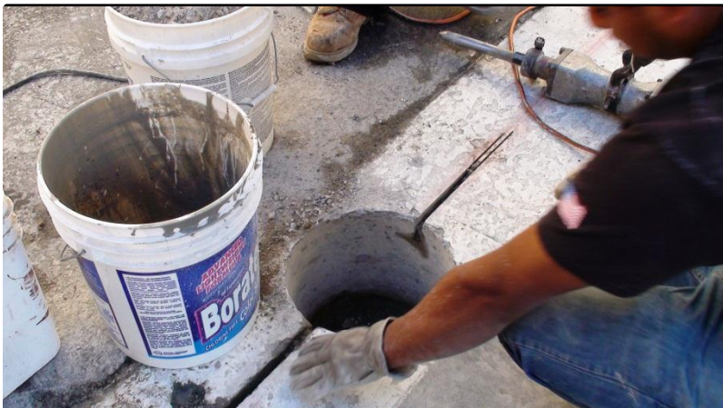
Figure 19: Into Each Hole, a Base Can is Mounted. The Base Can is Used to Stabilize and Protect the Fixture
