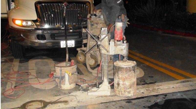
Figure 17: The Next Step in the Process is the Core Drill
