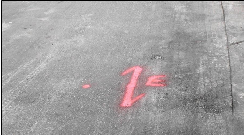
Figure 9: First Order of Business – Locate All Utilities and Mark with APWA Color Code, Red = Power Line
