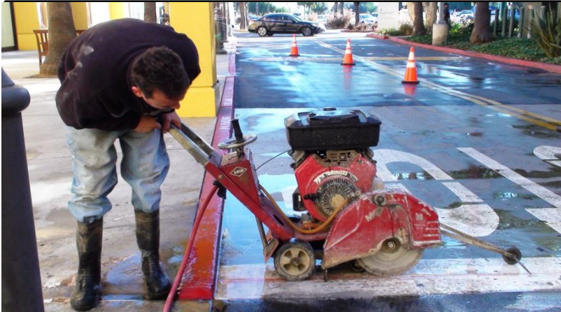
Figure 13: Once Fixture Locations are Defined Saw Cuts for In-pavement Wiring Can be Made
