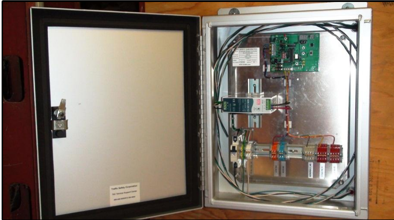
Figure 33: Field Wiring is then Connected to the Terminal Blocks in the Enclosure and the System Setup for Operation
