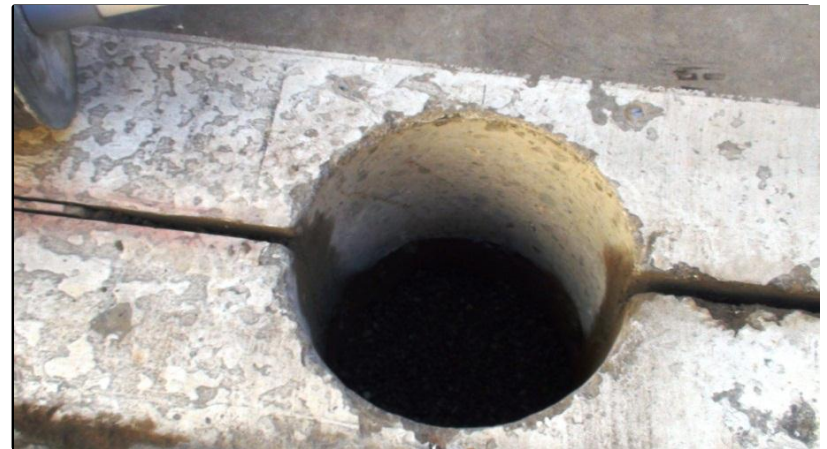
Figure 20: Once the Holes are Drilled, Gravel is Placed at the Bottom of Each Hole to Provide a Drainage Area
