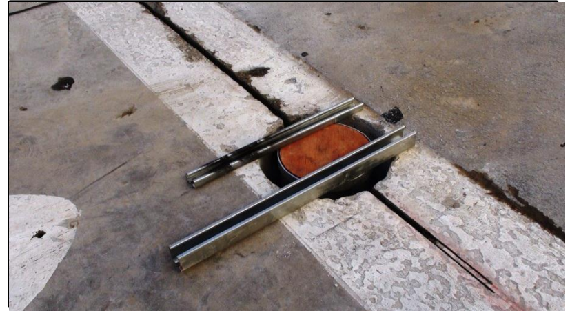
Figure 22: Base Cans are then Positioned to Align the Fixtures for Best Visibility by Drivers. Field Wiring is Inserted into the saw Cut and Concrete is Poured
