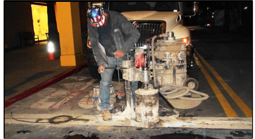
Figure 18: At Each Fixture Location a Core Drill is Made. Cores are Approximately 12" Dia. X 28" Deep
