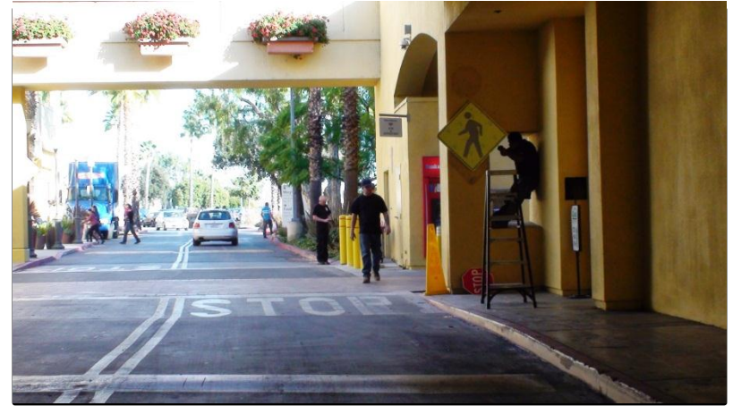
Figure 26: Pre-warning Signs are Mounted on Both Sides of the Crosswalk
