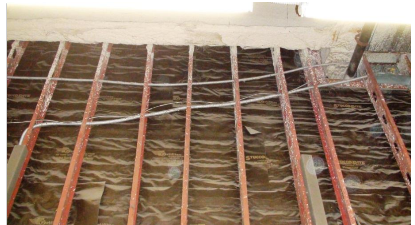
Figure 28: Wiring is then Routed Down to the Control Enclosure Mounting Location
