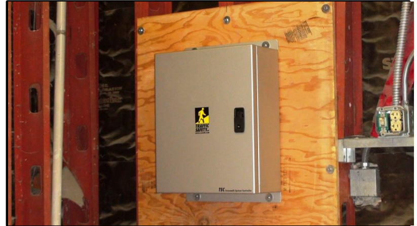
Figure 34: Controller Shown in NEMA 4 Enclosure
