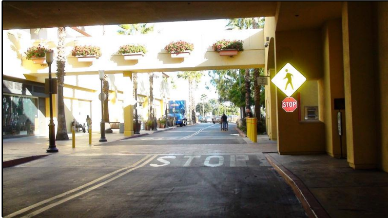
Figure 29: Once again, Wiring from the LED Edge Lit Sign is Routed Through the Column and Archway
