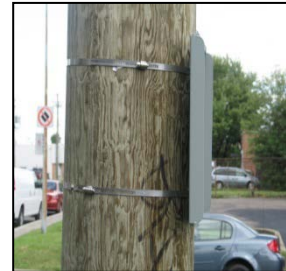
Figure 11: Profile view of Pole Bracket
