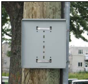
Figure 9: Pole Bracket banded to utility pole
