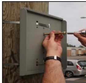
Figure 10: Additional lag bolts should be used for added security
