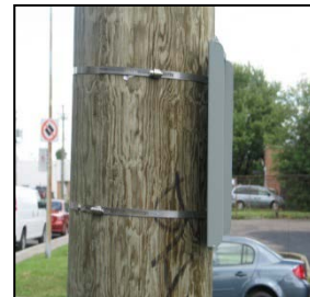
Figure 11: Profile view of Pole Bracket
