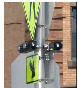
RRFBs are placed on both sides of a crosswalk in a single or double-sided (back-to-back) configuration.
