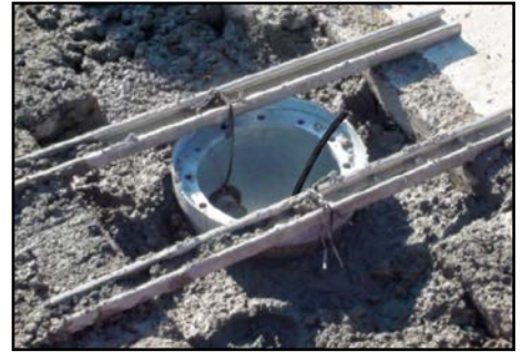
Base Can Installed in Roadway
