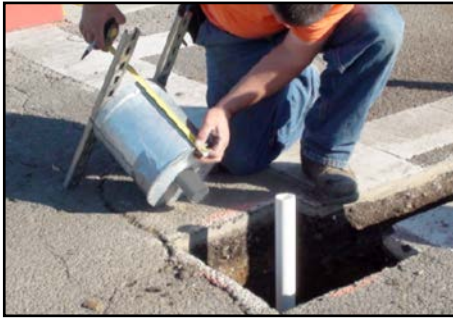
Mounting Jig Attached to Base Can
