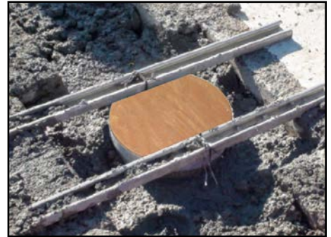
Base Can Installed in Roadway
