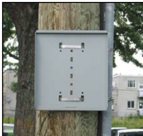
Figure 9: Pole Bracket banded to utility pole
