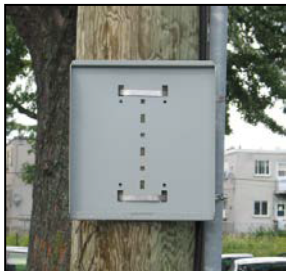
Figure 9: Pole Bracket banded to utility pole
