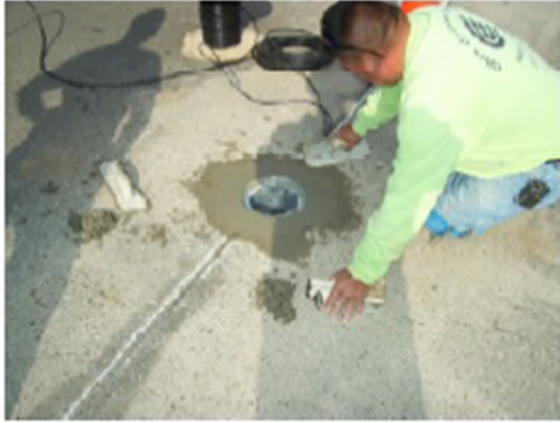
Base Can in Concrete
