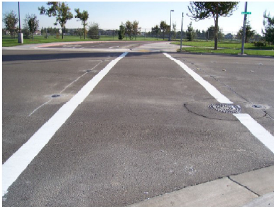
Fixtures Placed in Base Cans
