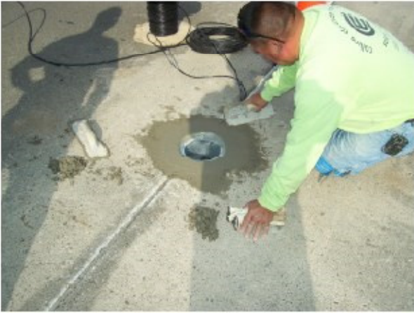
Base Can in Concrete
