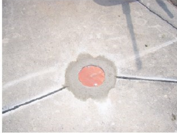
Plywood Protective Cover
