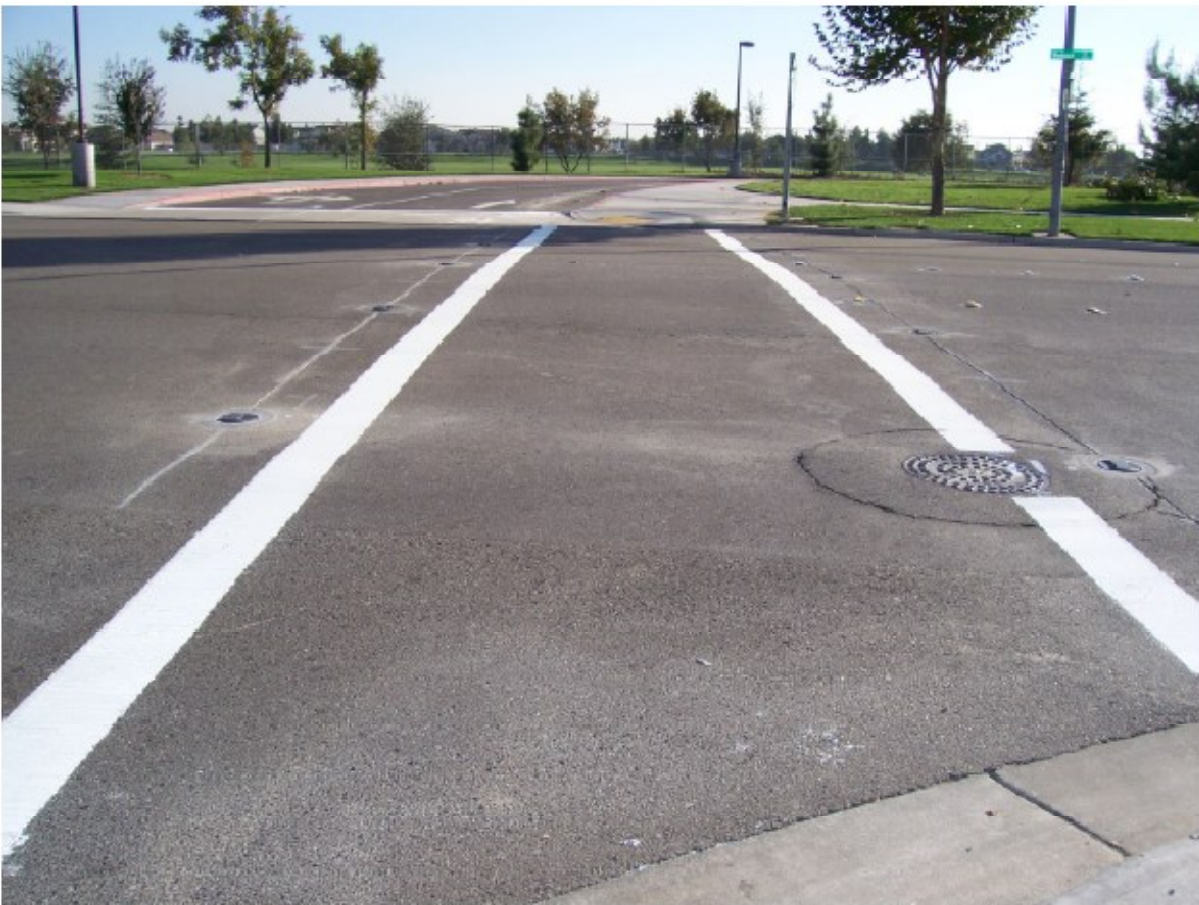
Fixtures Placed In Base Cans
