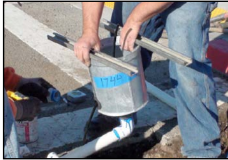
Base Can Attached to Drain Conduit
