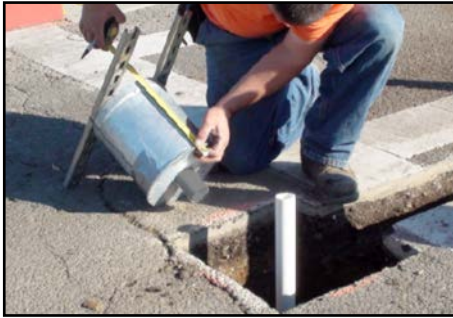
Mounting Jig Attached to Base Can
