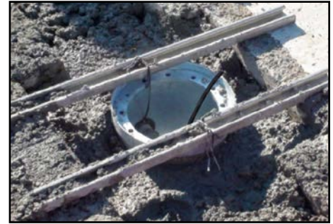
Base Can Installed in Roadway
