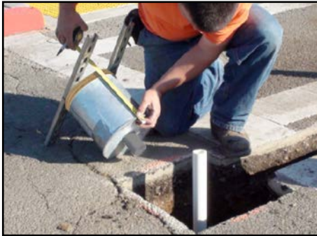
Mounting Jig Attached to Base Can
