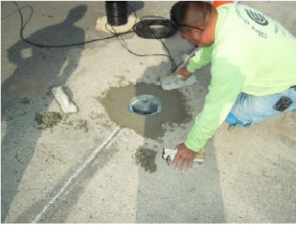
Base Can in Concrete
