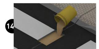
Introduce approximately 7.5Kg of SIKADUR 42 SP glue (or alternative glues \*) in the respective slot for the CROSSLED. This amount of glue can vary depending on the total area milled.
