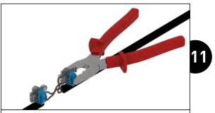
Use pliers to press the connector cover, in order to create the connection between the wires.
