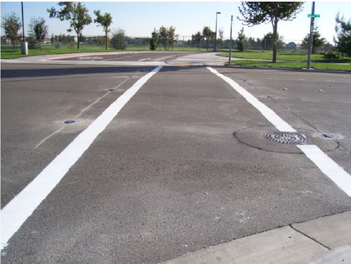
Fixtures Placed In Base Cans
