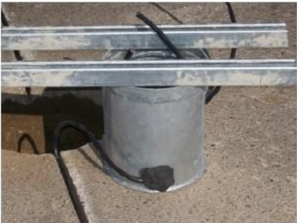
Mounting Jig Setup
