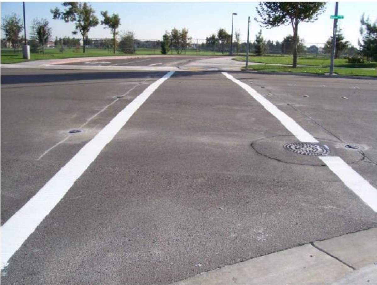
Fixtures Placed In Base Cans
