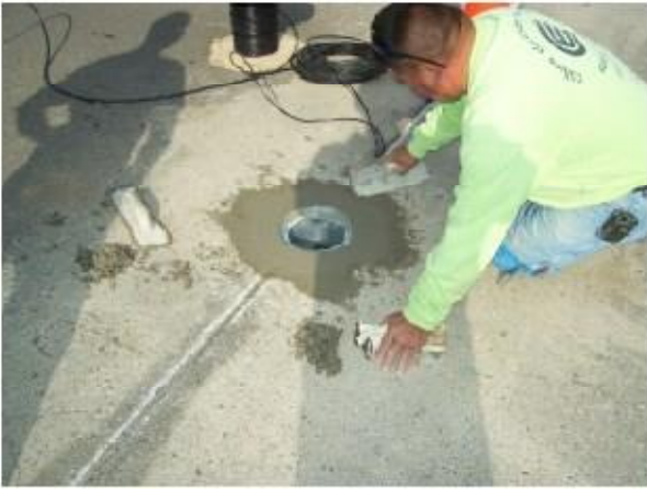
Base Can in Concrete
