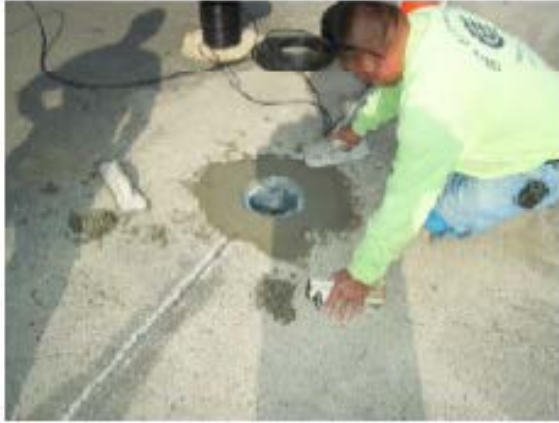
Base Can in Concrete
