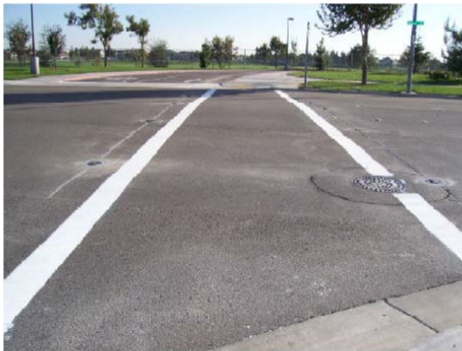
Fixtures Placed in Base Cans
