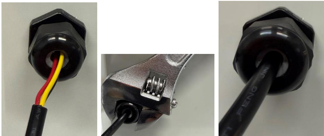
Solar Panel Cable Gland Installation
