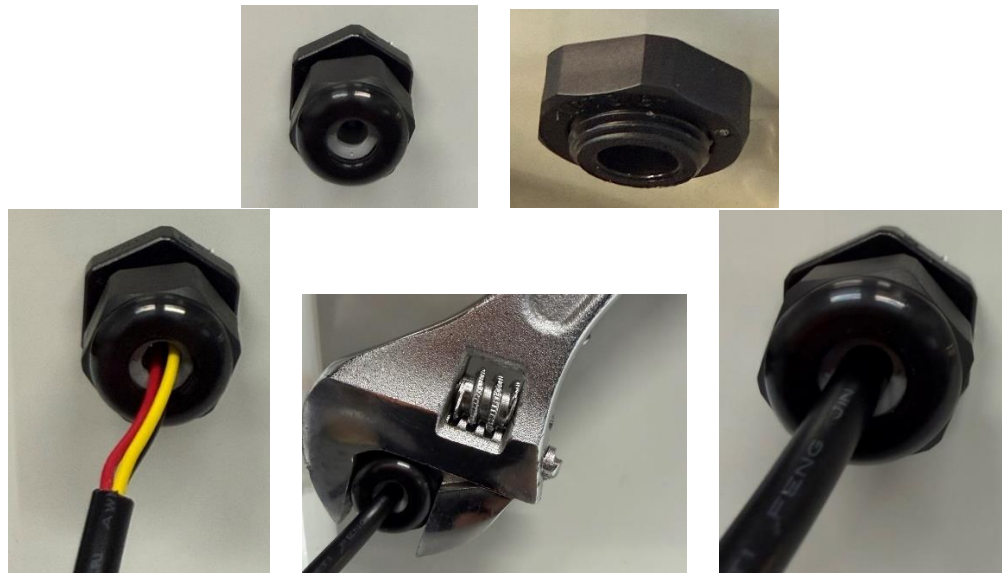
Solar Panel Cable Gland Installation
